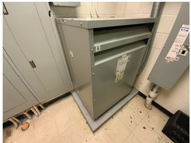
24 - SECONDARY TRANSFORMER
